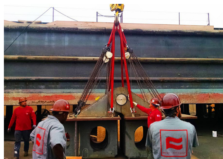
Hinge ready to be installed
