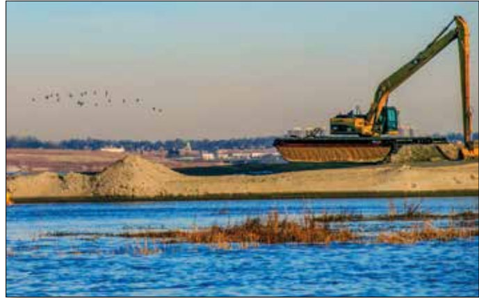
Sand used from the Harbor Deepening Program was used to remediate, restore and protect the marsh islands in Jamaica Bay, N.Y. (Photo USACE NY District)
