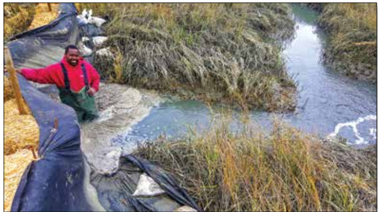
Crew member installing sediment barrier to contain 5 ft. deep water channel. Photo by Curtin Maritime
