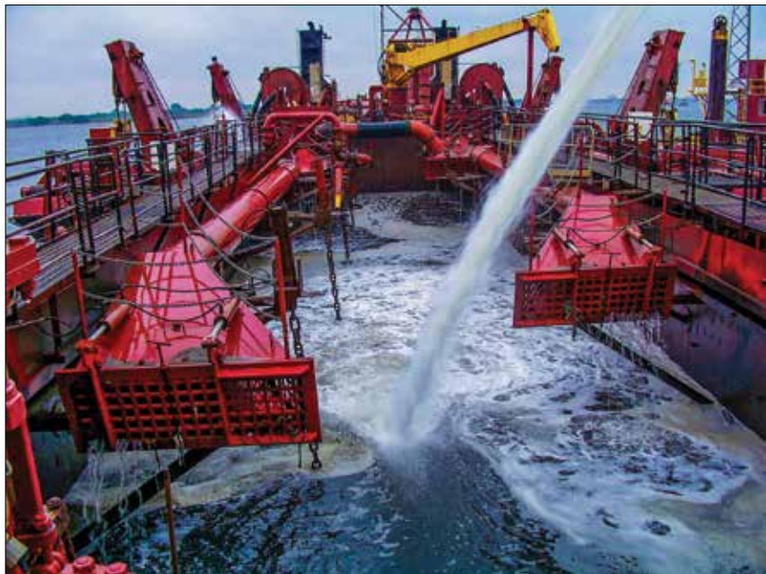
Sand being pumped at Jamaica Bay, N.Y. from the Harbor Deepening Program to restore marsh islands in Jamaica Bay, N.Y. (Photo USACE NY District)
