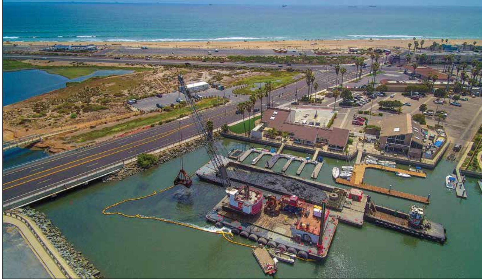
Derrick barge ( DB ) Ben Weston ( 150 t Lima 2400C4L Tier III ) dredging main channel east next to Pacific Coast Highway ( PCH ). Photo by Curtin Maritime
