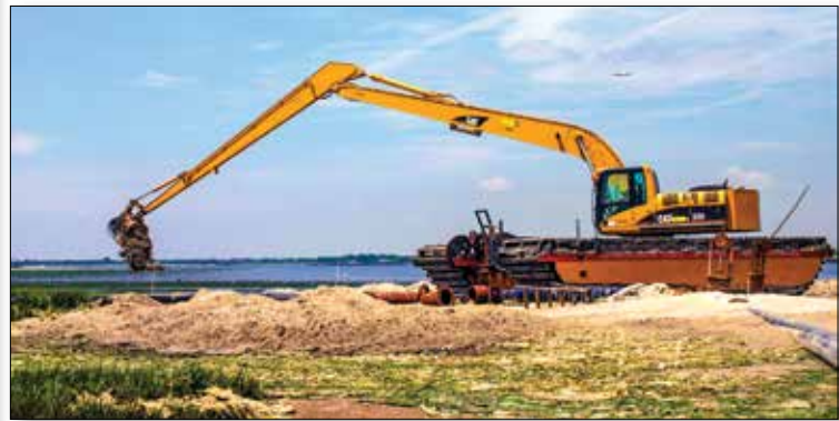
Sand being used from the Harbor Deepening Program to restore marsh islands in Jamaica Bay, N.Y. (Photo USACE NY District)
