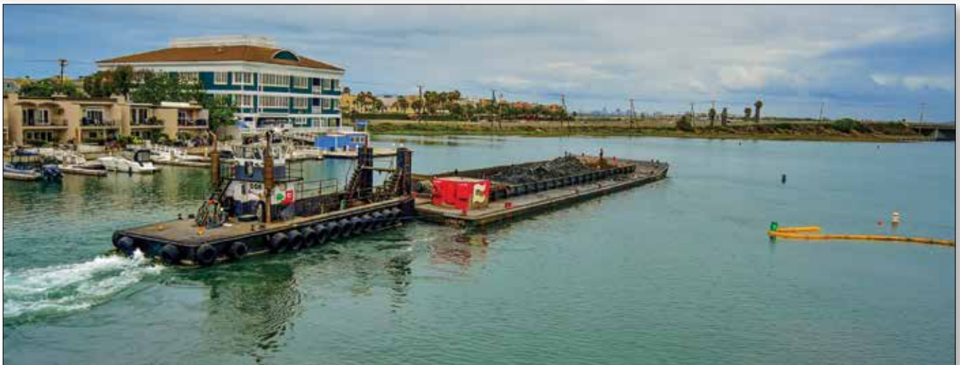
Main channel dredging depositing in the dump scow for transport.
