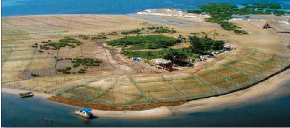
There was a considerable amount of engineering construction that went into the marsh islands construction at Jamaica Bay, N.Y.
