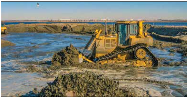
Sand being used from the Harbor Deepening Program to restore marsh islands in Jamaica Bay, N.Y. (Photo USACE NY District)
