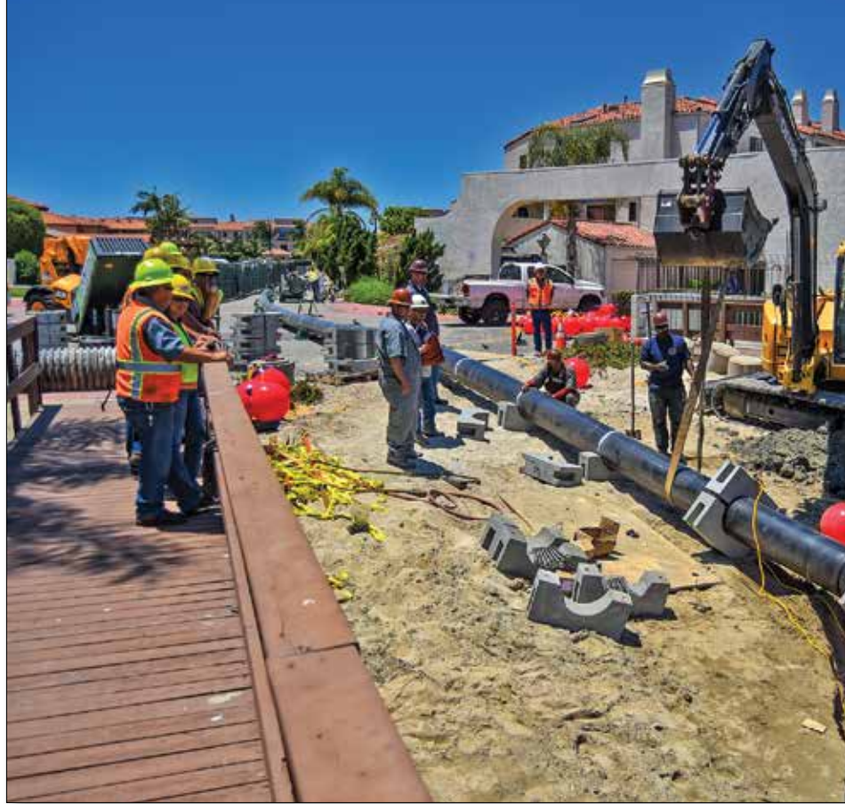
Installation of a 16" high density polyethylene pipe (HDPS) sub-sea waterline to provide critical infrastructure for the City of Huntington.
