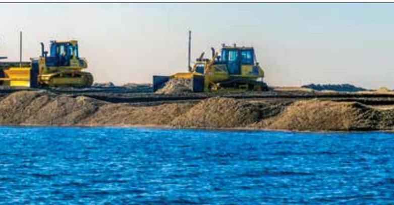
To quell further erosion of the islands, and adding to an already impressive list of habitat restoration projects in Jamaica Bay, the Army Corps placed millions of cubic yards of sand from the Harbor Deepening Program to restore marsh islands in Jamaica Bay. (Photo USACE NY District)
