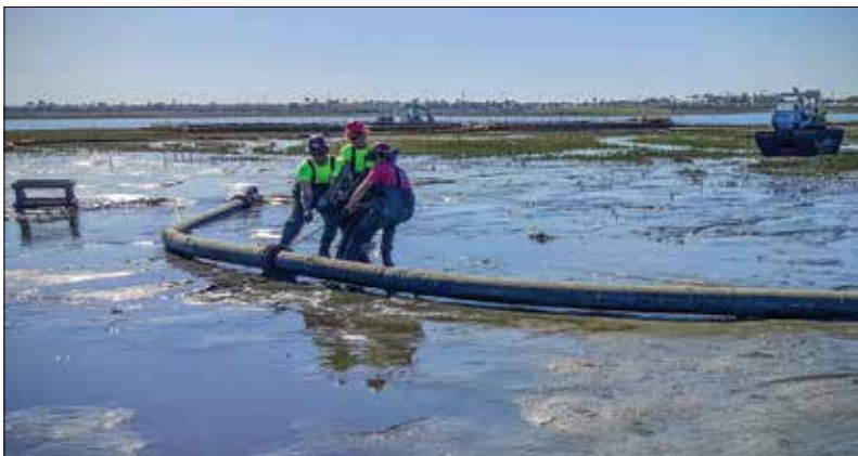
Maintaining placement pipeline. Photo by Curtin Maritime
