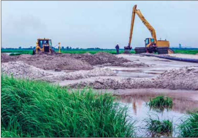
Sand being used from the Harbor Deepening Program to restore marsh islands in Jamaica Bay, N.Y. (Photo USACE NY District)
