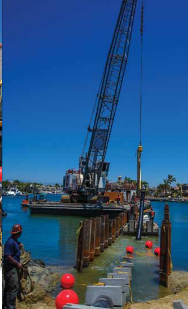
Installation of a 16" high density polyethylene pipe (HDPS) sub-sea waterline to provide critical infrastructure for the City of Huntington.
