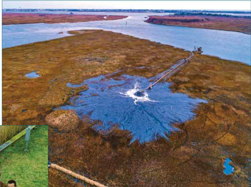
The U.S. Army Corps of Engineers and its contractor Barnegat Bay Dredging Company completed a dredging and habitat creation project near Stone Harbor, N.J. in December 2018. Work involved dredging a portion of the federal channel of the New Jersey Intracoastal Waterway and beneficially using the material to create habitat on marshland owned by the New Jersey Division of Fish & Wildlife. Credit: USACE.
